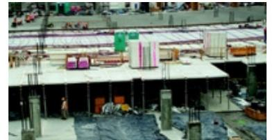
**On this congested inner-city site, workers are building the first below-ground parking garage level. In the background one-third of the deck is being finished while deck forms are being positioned for the middle third. Photo: Hensel Phelps**
