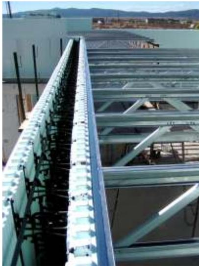
The second type of connection uses the TrusSteel TSUC clips. The clips are fastened to the concrete wall with Tapcon® fasteners and to the TrusSteel trusses with #10 self-drilling tapping screws. Several sizes of TSUC clips are available, depending upon the required load transfer capability. Refer to TrusSteel Standard Details TS030 and TS031 for a description of these connections as well as a chart describing the rated uplift resistance of each application.
