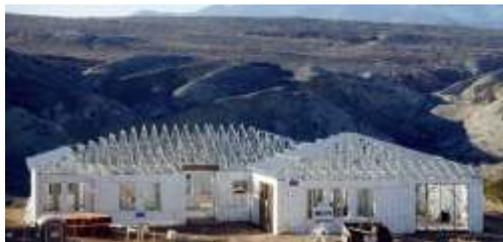
to the steel supports and fastened to the trusses with #10 self-drilling tapping screws, can provide resistance to large uplift reactions. Refer to TrusSteel Standard Details TS027 and TS027A for installation requirements and connection capacities. (Editor's Note: You can also find this information in Section 5 of the new Truss Design Manual).
